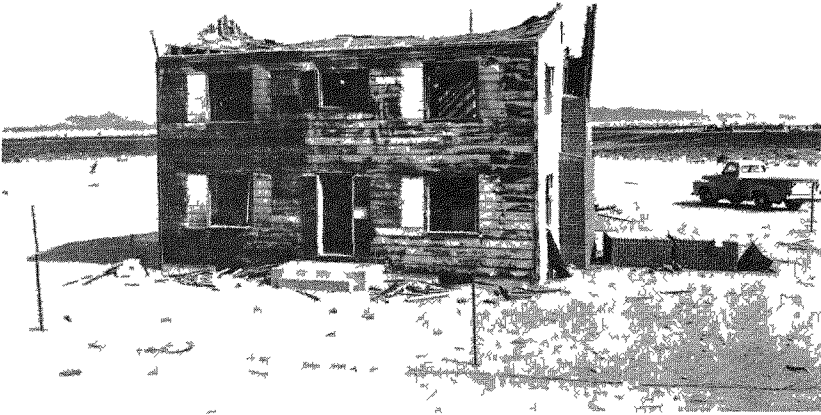
Figure 4.22 Strengthened wood frame house after a nuclear explosion (4 psi overpressure)
